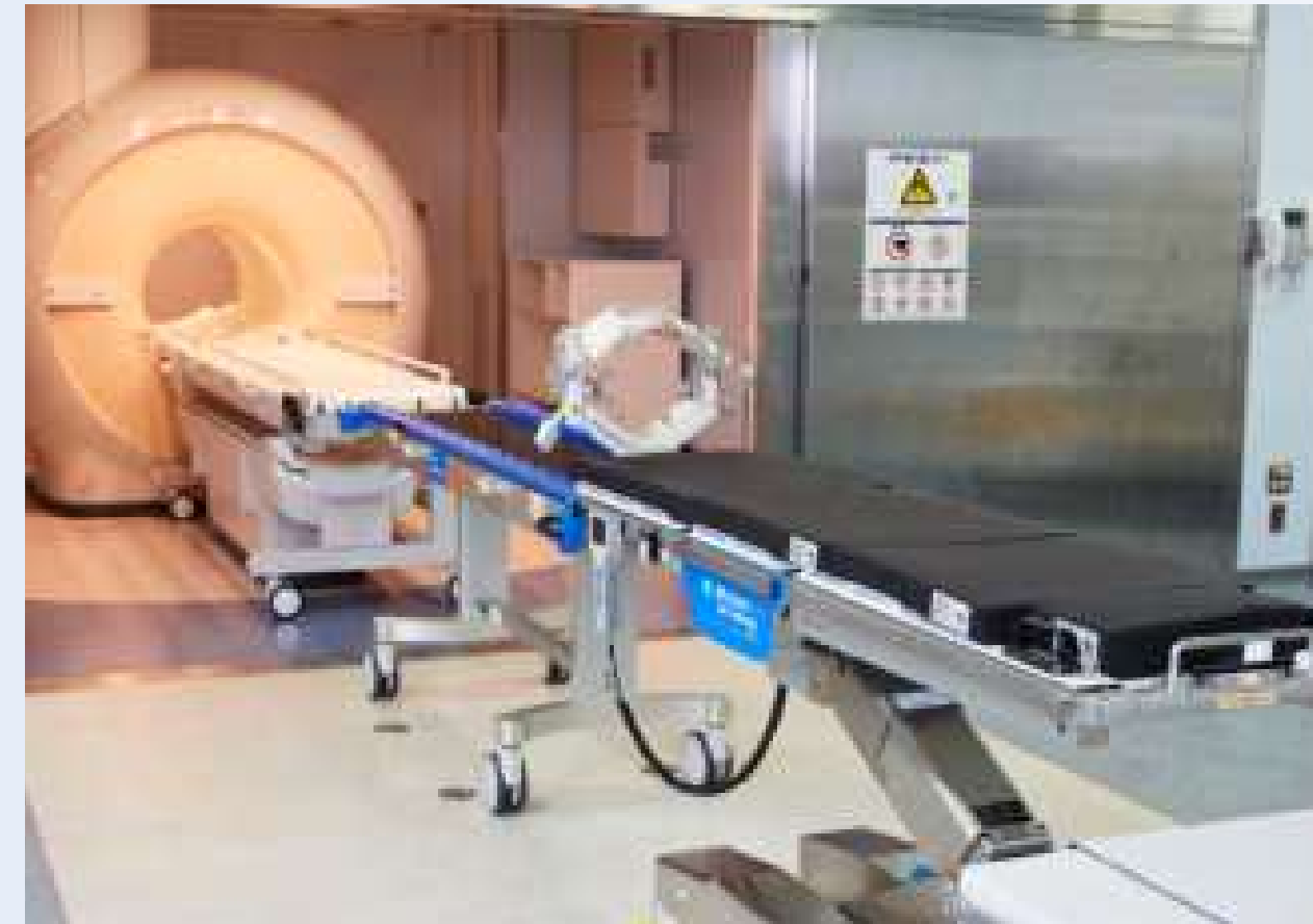
Layout of the intraoperative MRI suite as part of the MXRO suite.
